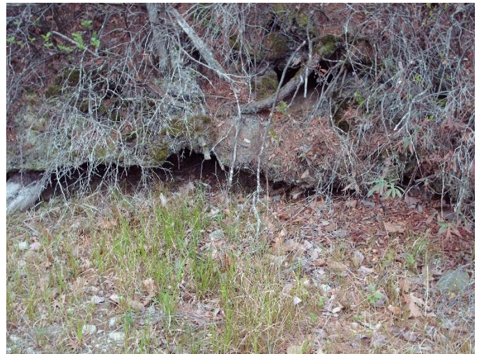
Undercut banks observed at Downing Pond during a drawdown. Photo credit Fred Quimby.
