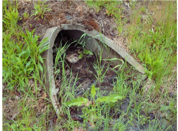
One of several stormwater drainage outfalls from Route 11 to Mill Pond that tested high for total phosphorus. Detailed assessment of the stormwater drainage network in this area will help identify appropriate management actions.
